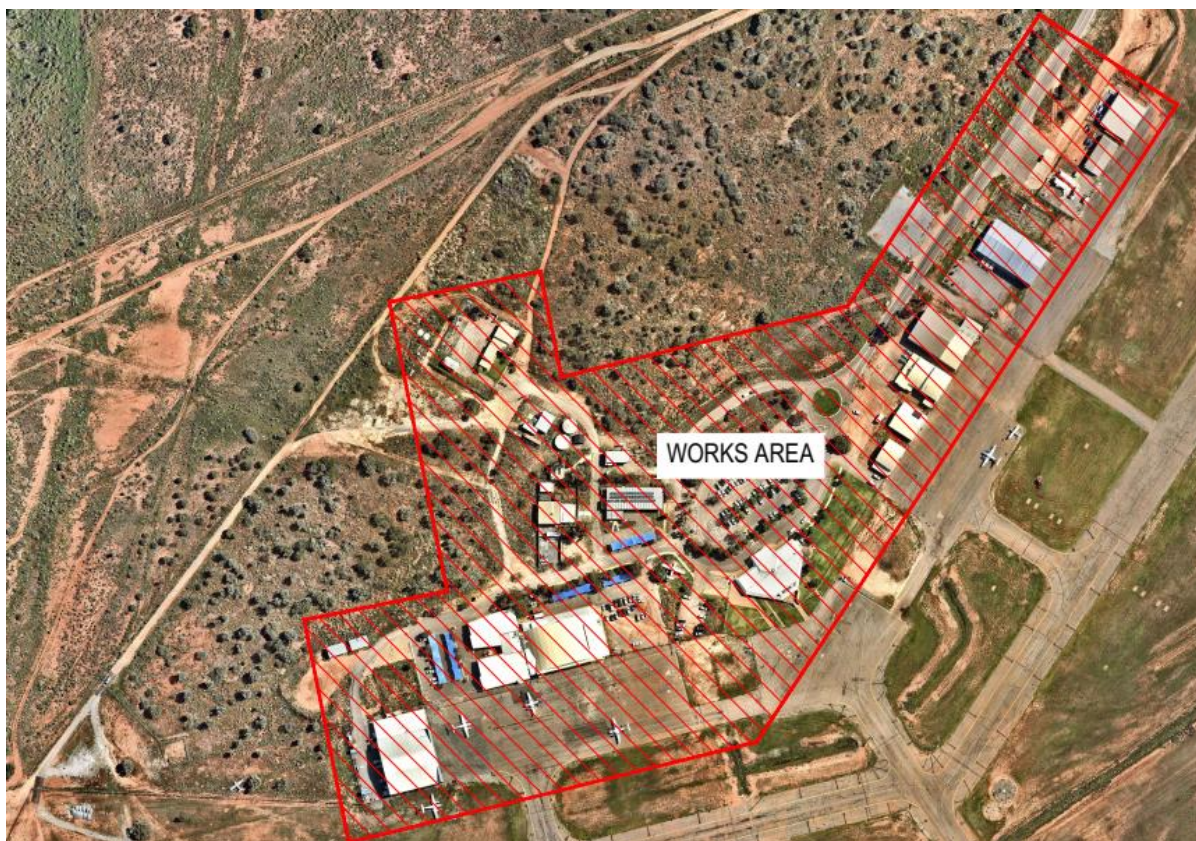
Extent of the works area – GHD Pty Ltd
