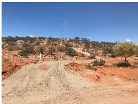
Image: Construction of new campsite walking trail.
