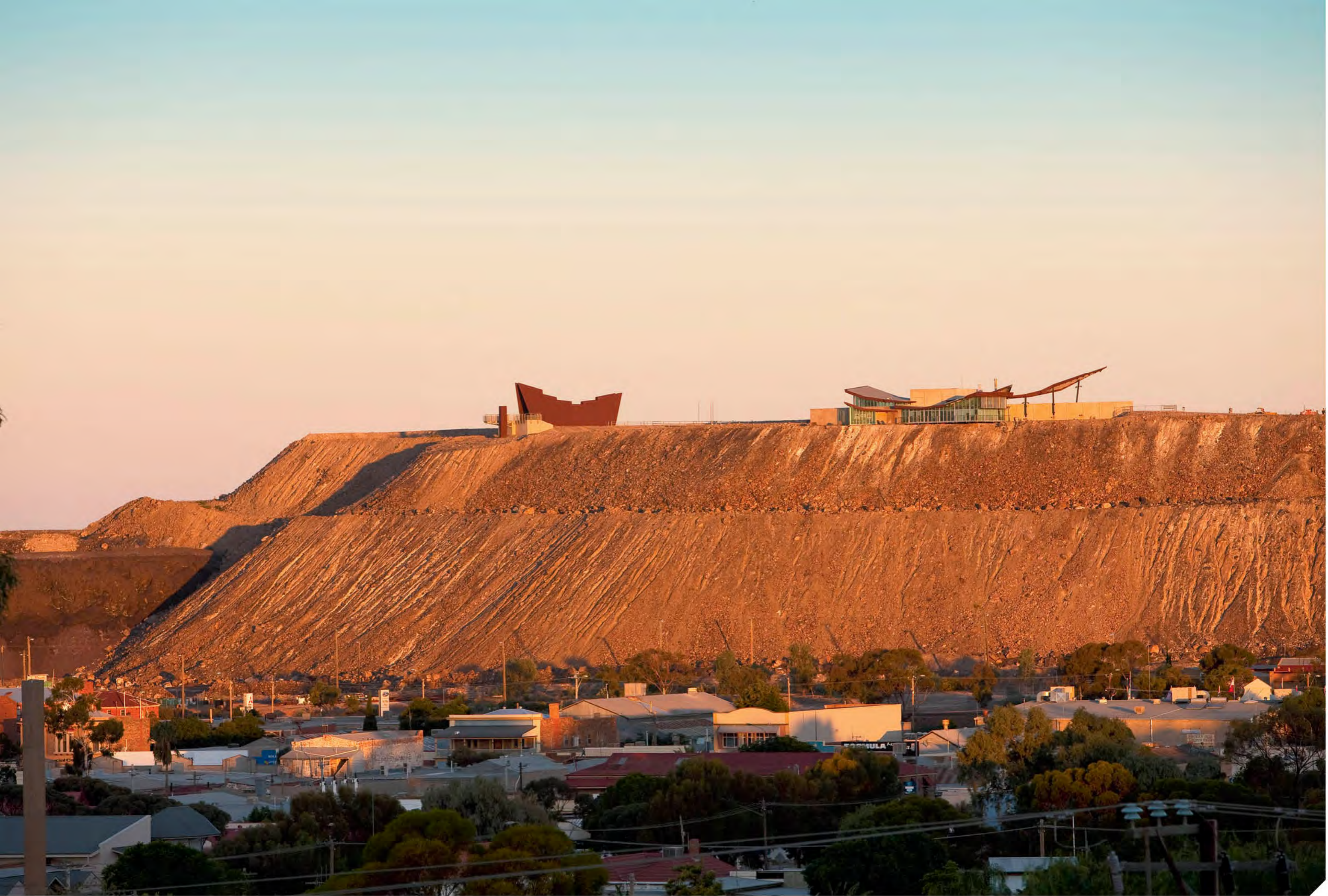
Above: The Line of Lode Miner's Memorial is an iconic piece of architecture that sits proudly above Broken Hill.
